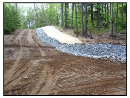
Camp road undergoing reconstruction. Road has been regraded to direct runoff to rip rap drainage ditch / detention structure along road side and new grass strip has been installed for soil stabilization.
