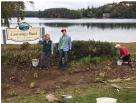
Maintenance of stormwater landscape features is very important. In partnership with the town of Bristol and community volunteers, our Youth Conservation Corps has worked to maintain the Cummings Beach stormwater swale for the last three years.
